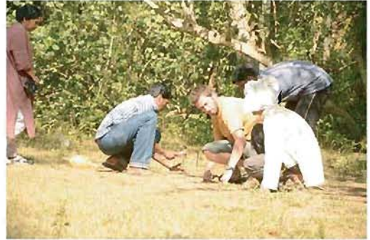
Laying out the trenches
